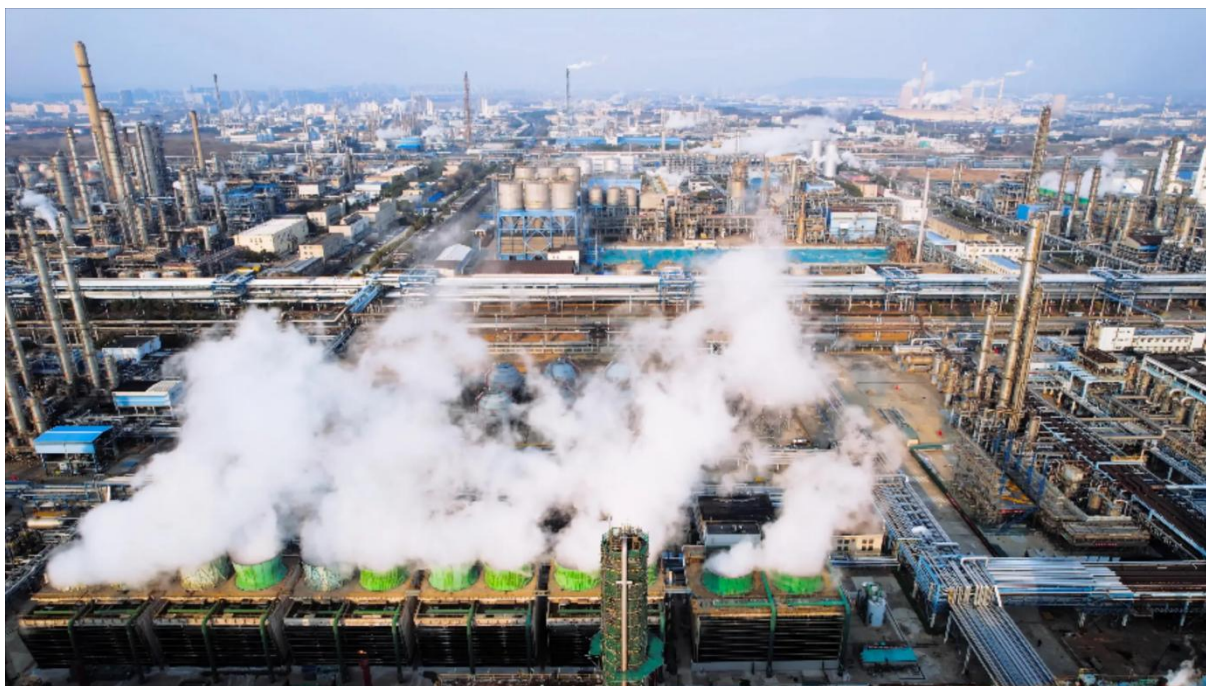
A typical large-scale chemical / petrochemical complex — a core market segment served by Filtearth fiber bed mist eliminators.
